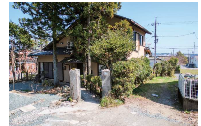
⑤ 到着です、この門柱が入口です Arrived, this gatepost is the entrance
